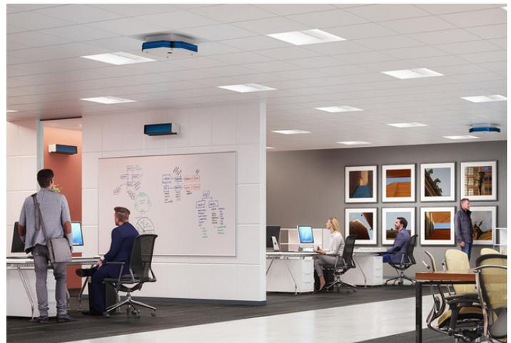
**Photo 1.** This office space uses two types of upper air GUV luminaires. The ceiling-mounted and wall-mounted units are located well above a 7-ft height for safety.
